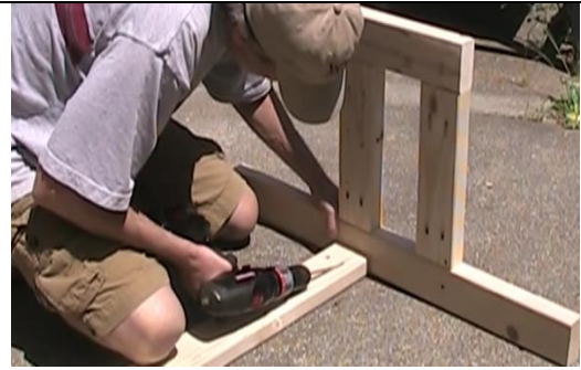
Fastening the wooden structure with drilling screws
