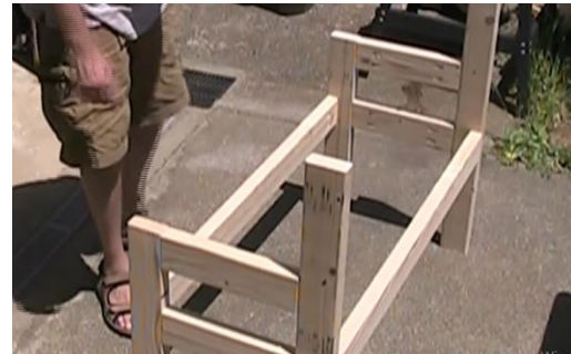
Installation of bench supports with a drill
