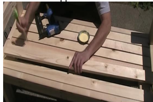
Bench seat installation
