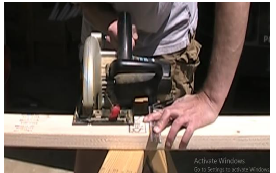
Cutting the wood according to the predetermined size
